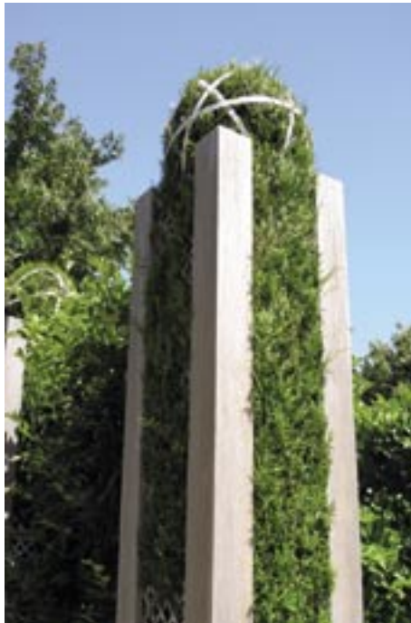
A botanically 'primitive' conifer is the 'round thing' within a four-square made from 215mm baulks of Irioko wood. It is a Garden-Architecture that rotted after 25 years.
